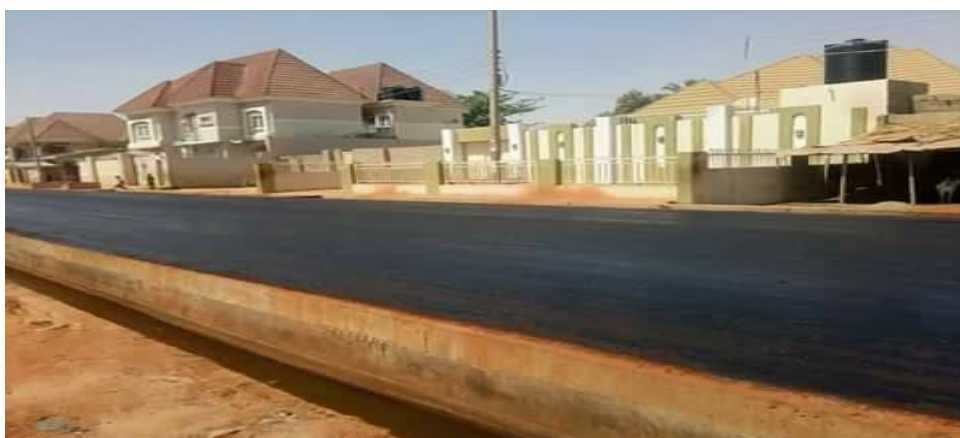
Figure 5. Newly Constructed Hadejia Town Ship Roads June 2018.
