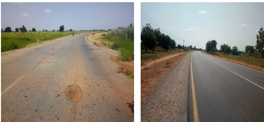
Figure 8. Old Dilapidated Tasheguwa- Road in 2015 Newly Renovate Tasheguwa-Guri Road 2018.
