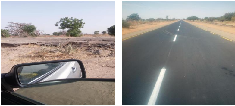
Figure 7. Old Dilapidated Kwanar Dundu, Bulangu Road 2015 Newly Re-constructed Kwanar Dundu Bulangu Road June 2018.
