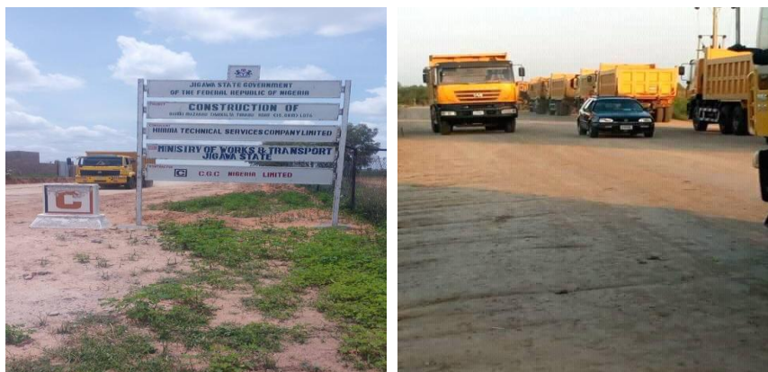
Figure 6. Hadejia, Garin Mutum Daya, Turabu Road Under Construction.
